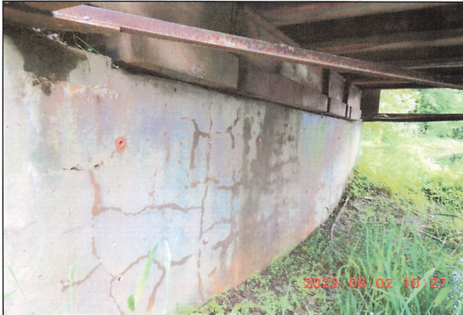
Photo 7: West Abutment Wall
