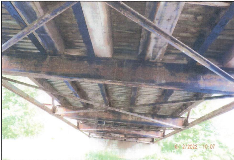
Photo 5: Interior Soffit, Stringers, and Floor Beams Looking West
