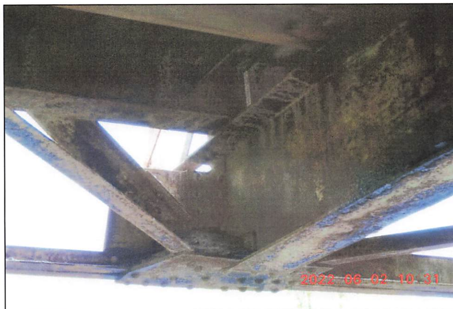
Photo 10: Typical Bottom Chord Floor Beam Connection
