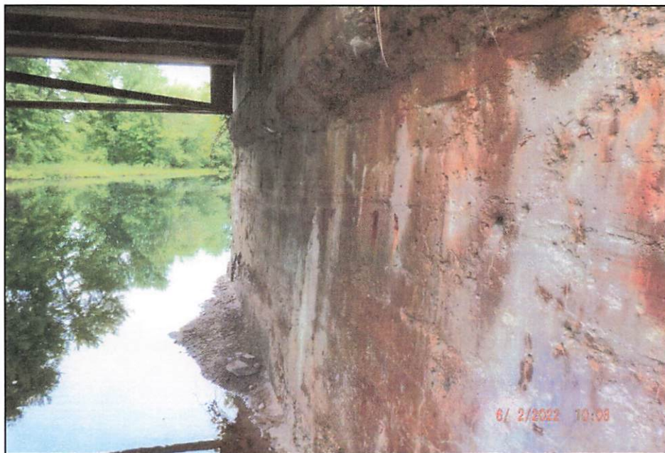
Photo 4: East Abutment Wall
